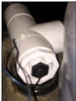
Sensor Installed in bulb well
